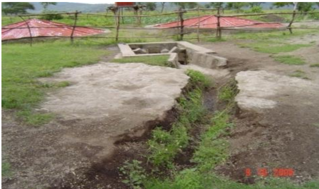
Photo 4.1 Underground rainwater tank in Siraro district. Credit: H. Nega, MoA
