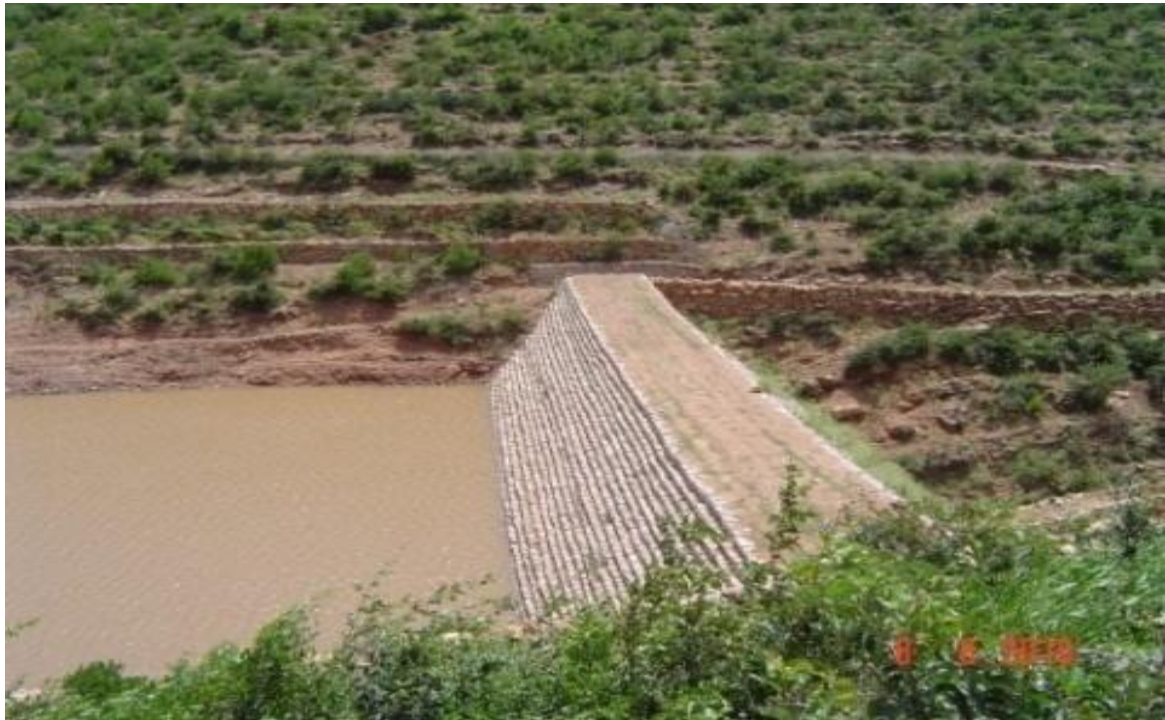
Photo 4.5 Sediment storage dams in Dire Dawa Administration. Credit: H. Nega, MoA
