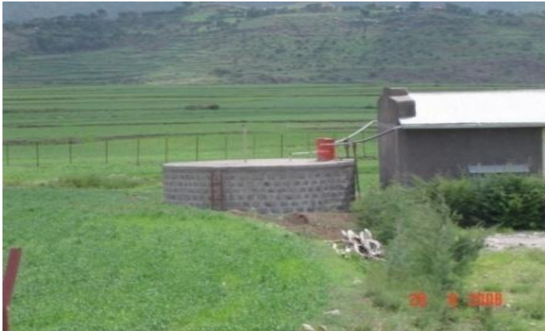
Photo 4.6 Rooftop rainwater harvesting in Tigray Region. Credit: H. Nega, MoA
