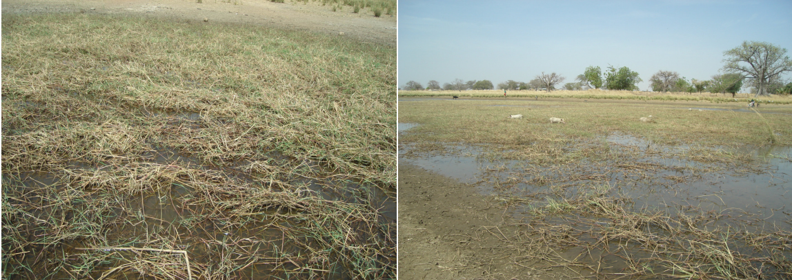
Figure 8 : Winkogo dam with reeds on the surface of the reservoir
