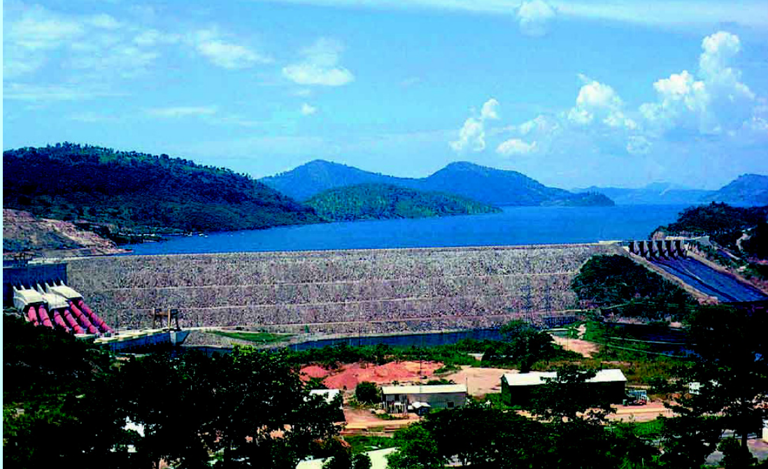
Photo: The Akosombo dam
