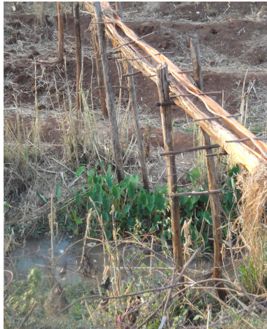
WATER DIVERSION CANALS IN MADA JALALA SMALL SCALE IRRIGATION SYSTEM INCLUDING THE WATER SUPER-PASS (FLYOVER) OVER THE RIVER BANKS IN THE MIDDLE (PHOTO BY BHARAT SHARMA, BIRHANU Z)
