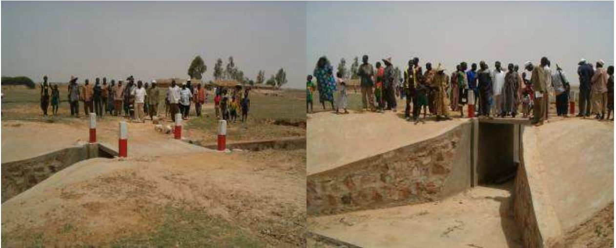
Photo 4.18. The gate of the Débaré after rehabilitation by the community
