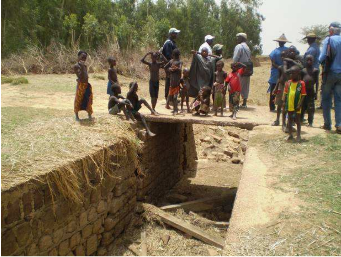
Photos 4.17. The initial poor condition of the sluice gate controlling the entrance and exit of water in and out of the Débaré pond (Batamani community) before CP72 intervention
