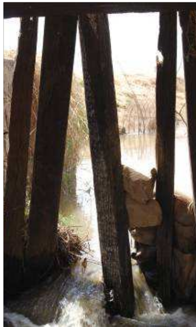
Photos 4.17. The initial poor condition of the sluice gate controlling the entrance and exit of water in and out of the Débaré pond (Batamani community) before CP72 intervention
