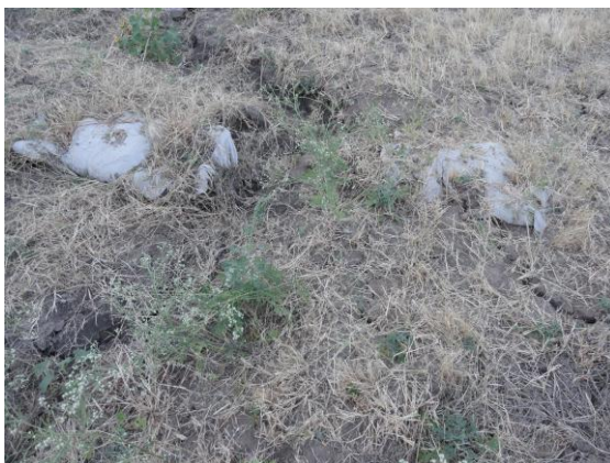
c. Sacs filled with sand and put on young gullies to protect erosion (effort made by one farmer around the study area).
