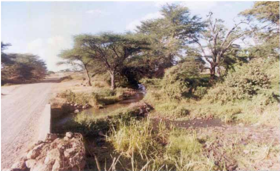
Plate 2. Simple water diversion weir at the Isinet bridge.
