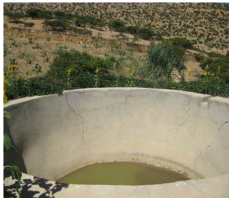
Underground tank is water empty
