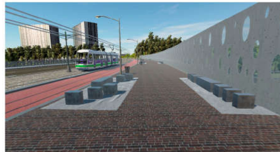
V4 - Whimsical S4 - 3m barrier: LAeq reduction 12.4 dB
