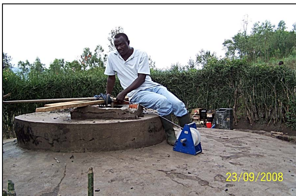
Figure IV.5. Measurement of the dynamic water level during the pumping test
