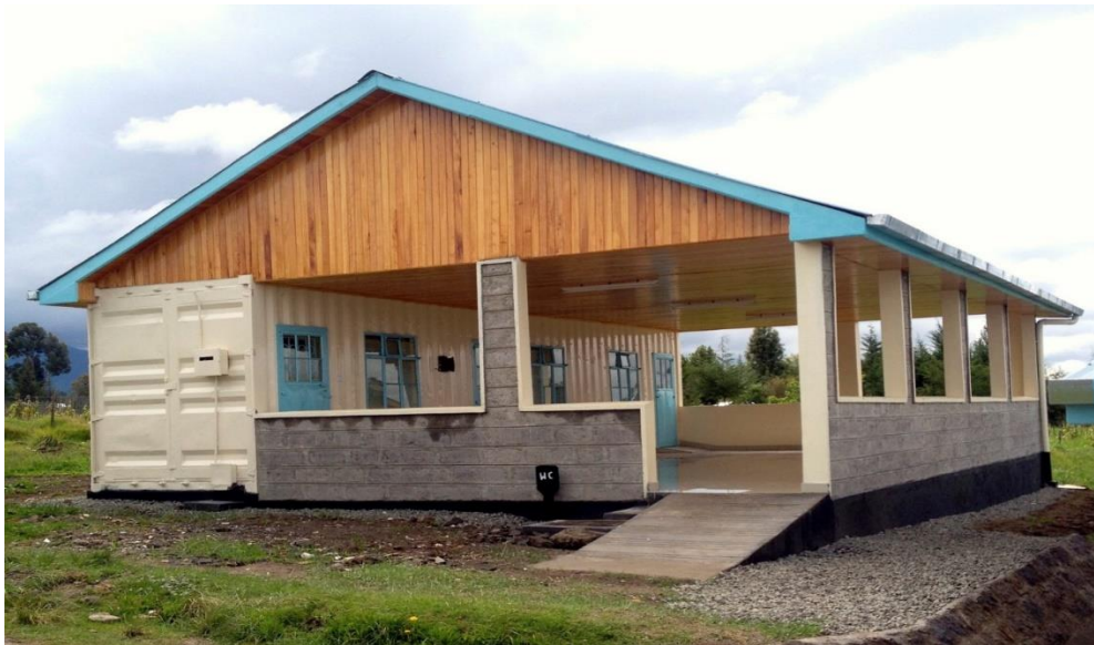
Figure 2.4 A House Created by Modifying a Container (Eco Homes Limited, 2016)
