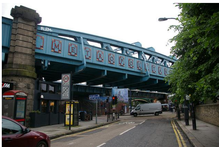
Figure 6. Kilburn High Road railway bridge. Source: Flickr, The Creative Commons.
