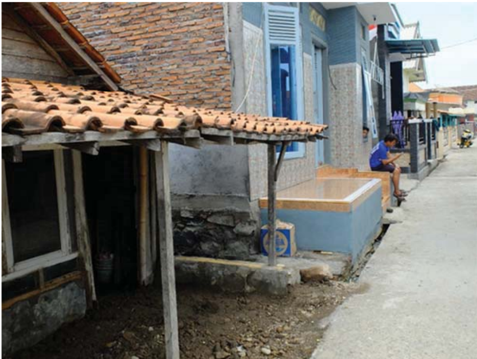
Fig. 4: The difference between the heightened house and the “sinking” house is evident, the community road has been renewed
