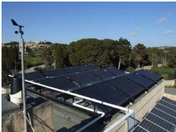
Figure 8: Vacuum tube solar collectors on the left and PV panels on the right.
