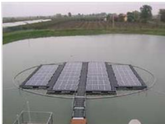
Figure 7: System at Solaralo, Italy. (From: http://www.luceonline.it/web/en/ricerca/costruzione-del-primo-impianto-fotovoltaico-galleggiante-in-puglia/ )
