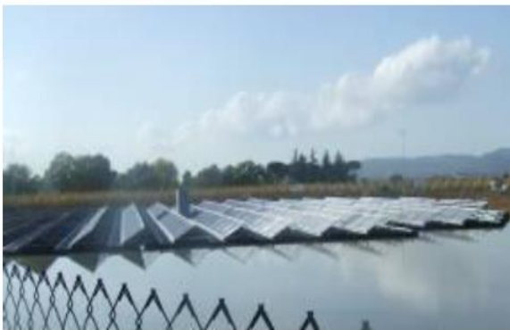
Figure 3: Setup in the Suvereto installation where the panels are installed at the optimal inclination with reflectors in front of them. The whole platform rotates to track the sun's position [4].
