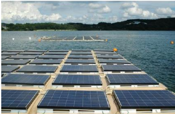
Figure 6: System in Aichi, Japan. 2x 10kWp, one water cooled. [7]
