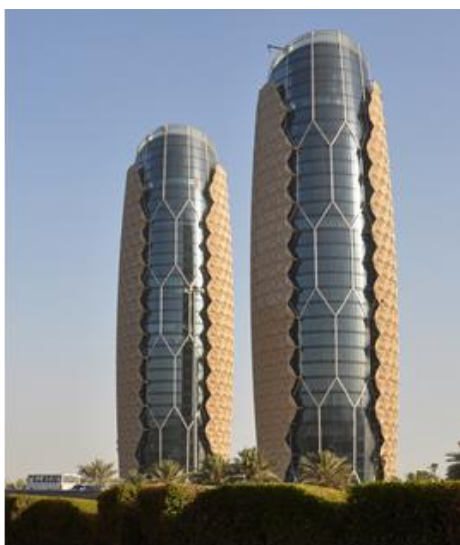
Figure 1: View of the towers from the North
