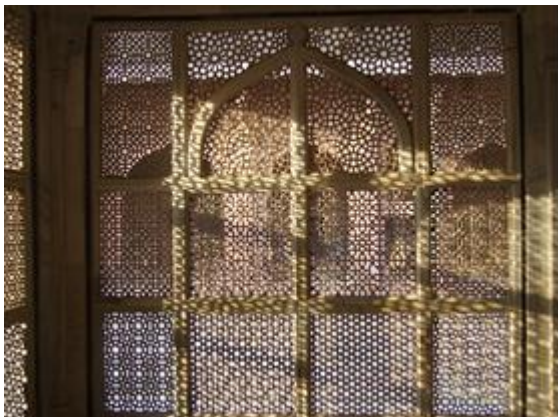
Figure 3: Traditional shading screens used in vernacular Islamic architecture
