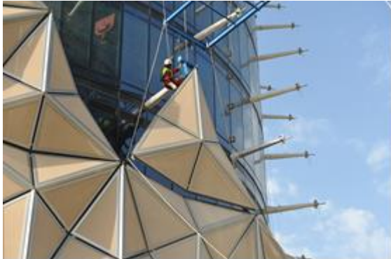
Figure 5: Mashrabiya installed onto supporting steelwork
