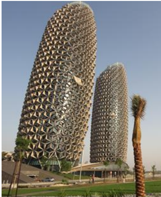
Figure 17: View of completed towers
