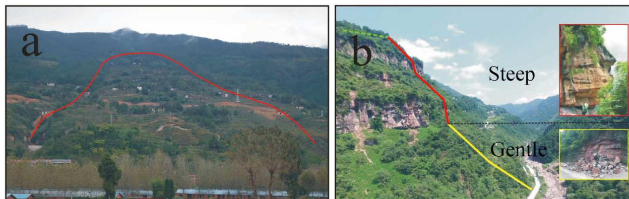
99 100 Fig. 2 Landslide types: (a) Colluvial landslide, (b) Multi-stage rockfall
