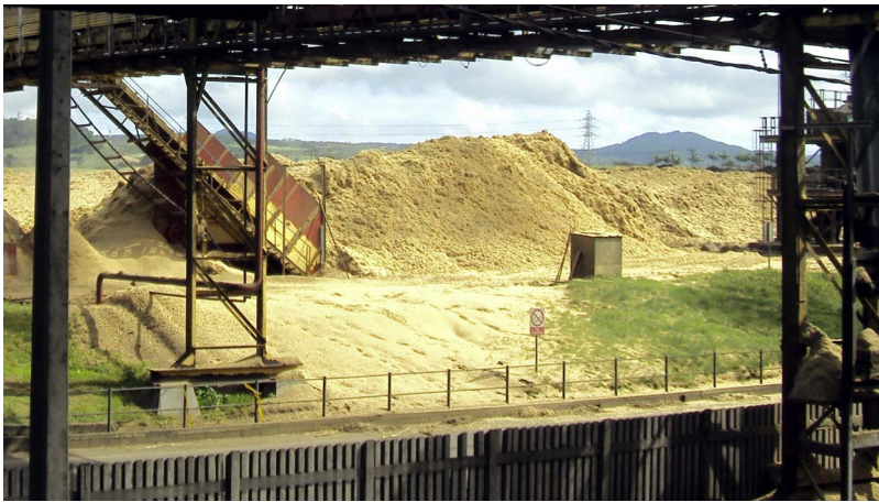
Fig. 1. Bagasse storage facility in Mauritius.
