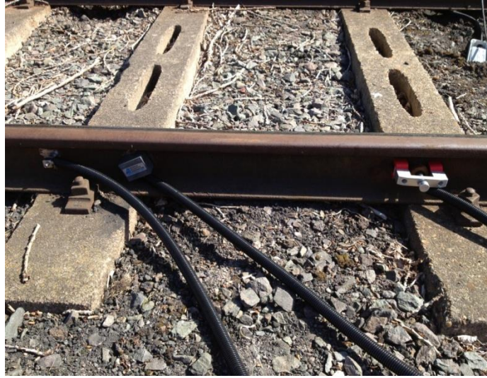
Figure 6-11: Photograph showing a pair of acoustic emission sensors together with an accelerometer mounted on the rail web at the Long Marston test track.
