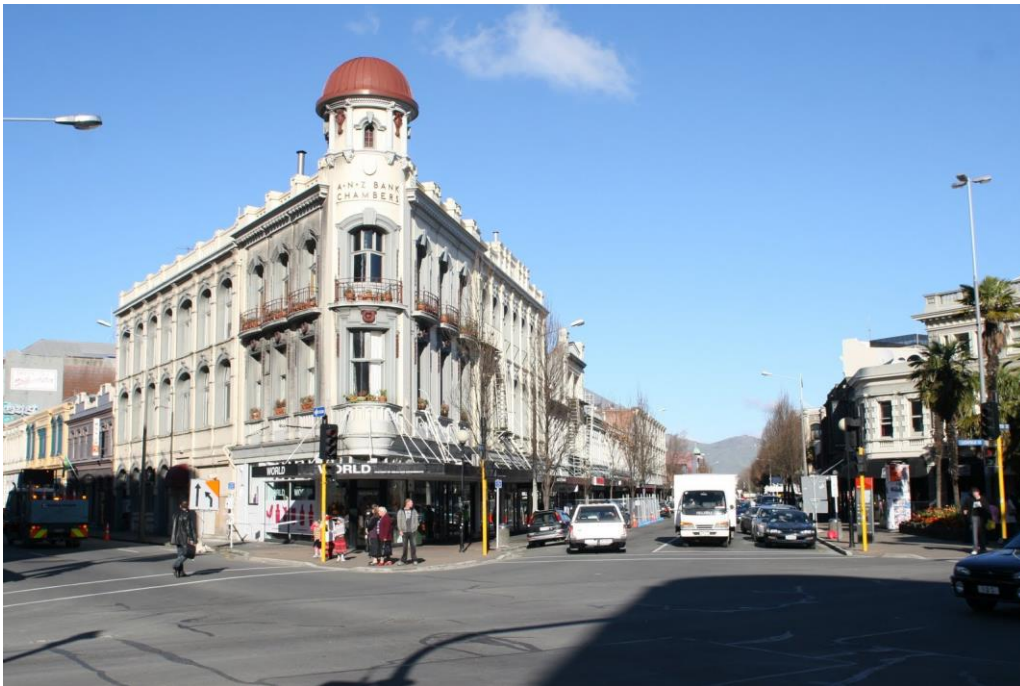
Figure 2.6 Former ANZ bank building pre- earthquakes (Source: http://2.bp.blogspot.com/ 8-DyTsoQSeI/TInoFbri-1/AAAAAAAAAPtg/n3JgIjoVLB0/s400/Copy+of+IMG_5187. )
