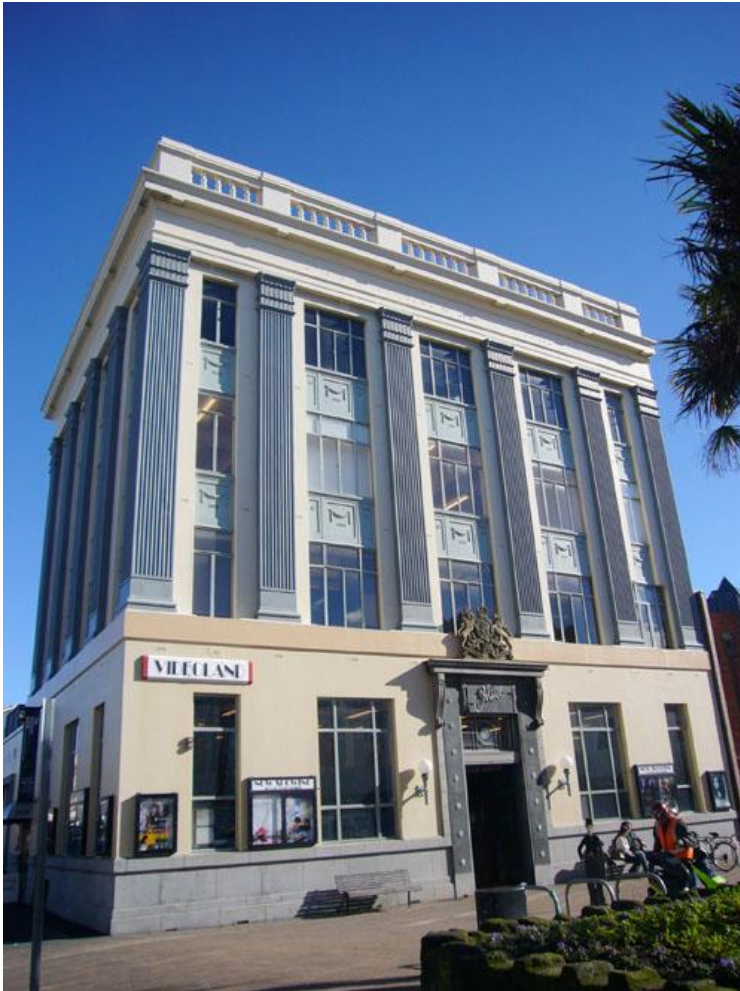
Figure 2.8 Former Post Office building pre-earthquakes (Source: Adrienne Rewi http://4.bp.blogspot.com/_yWEyPv7fm-/SJPeBqkw54I/AAAAAAAAABok/108BTn0x1d8/s1600/HiStPostOffice.jpg )
