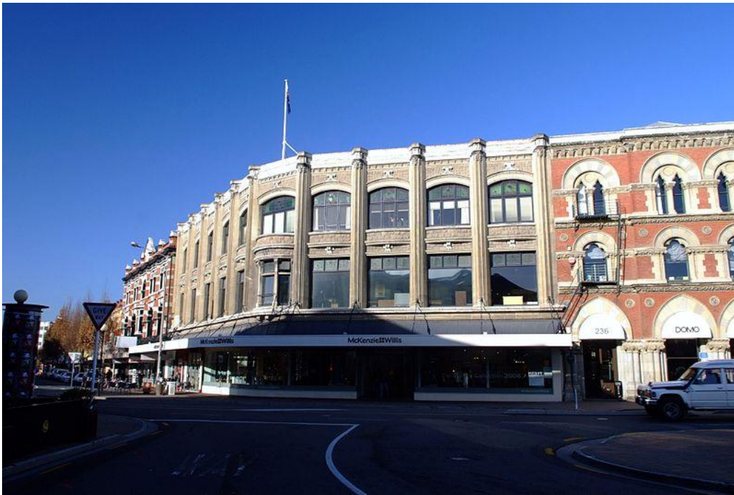
Figure 2.4 McKenzie and Willis Building pre- earthquakes June 2008 (Source: Francis Vallance https://commons.wikimedia.org/wiki/File:McKenzie_%26_Willis.jpg )
