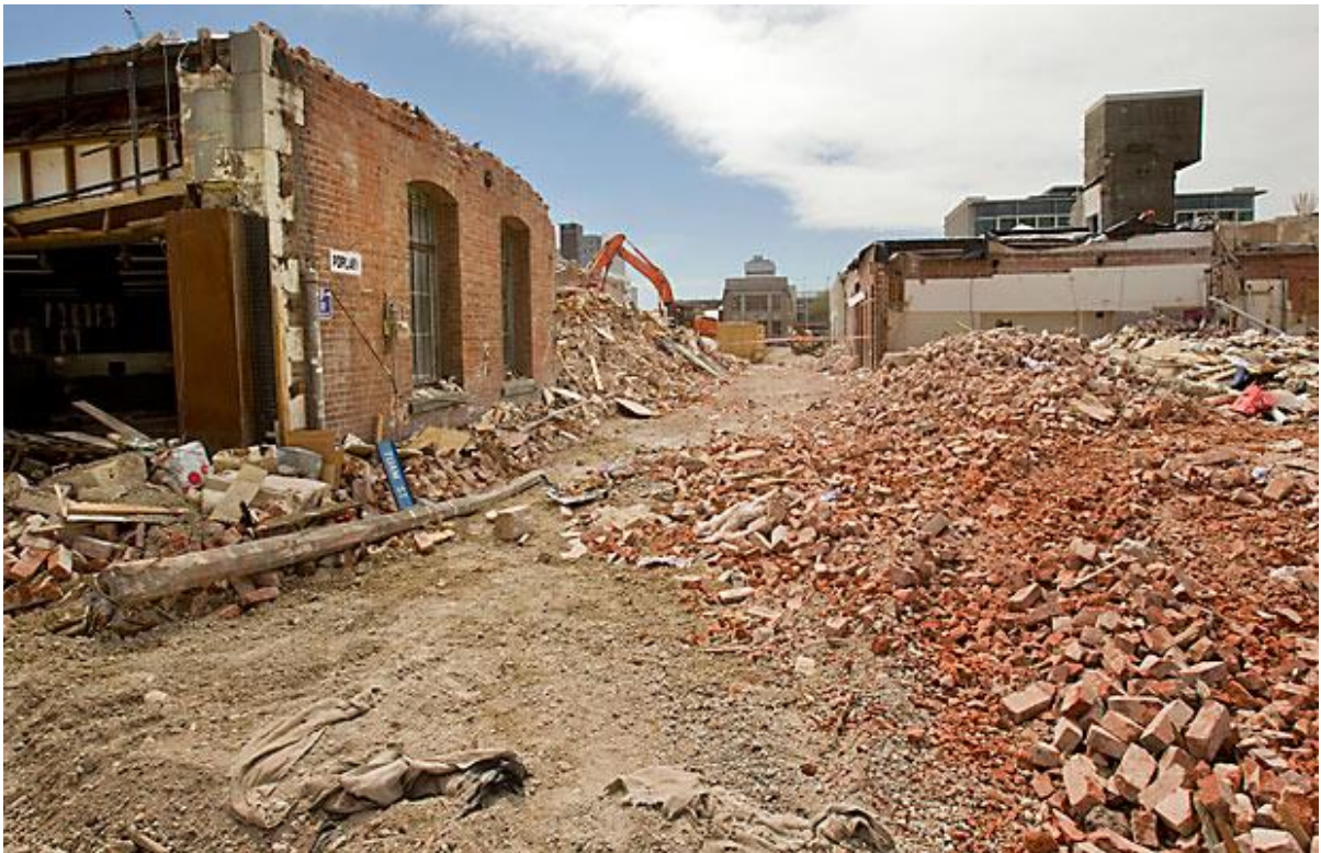
Figure 1.10 Poplar Street Looking south - demolition underway (Source: https://static2.stuff.co.nz/1328817776/202/6396202.jpg )
