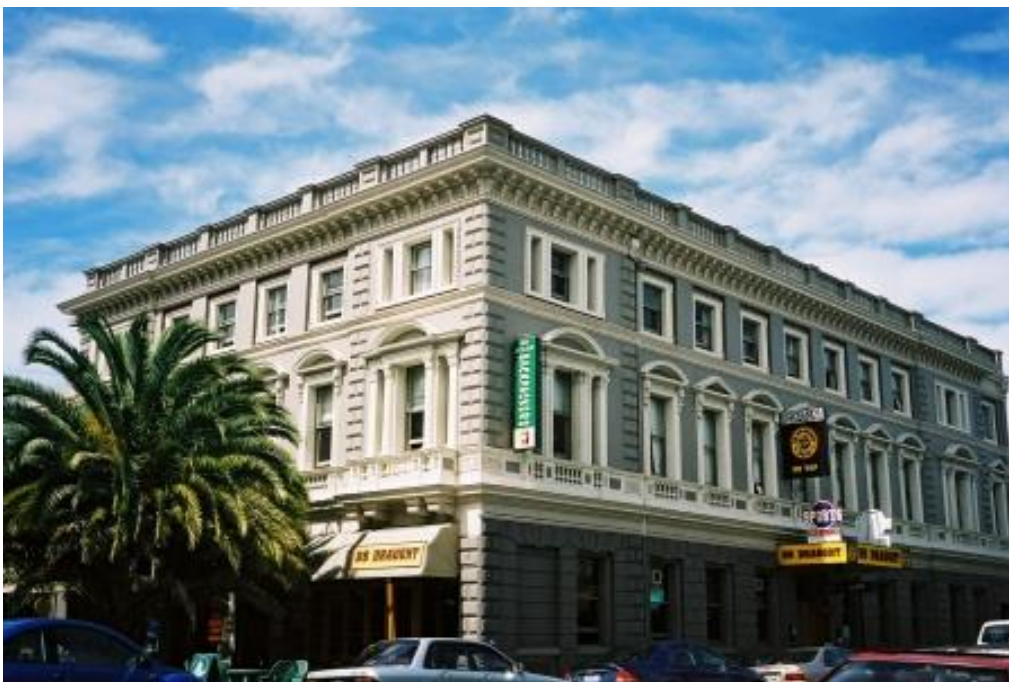
Figure 2.7 Excelsior Hotel building pre- earthquakes (Source: Heritage New Zealand http://www.highstreetstories.co.nz/stories/90-the-excelsior-hotel )
