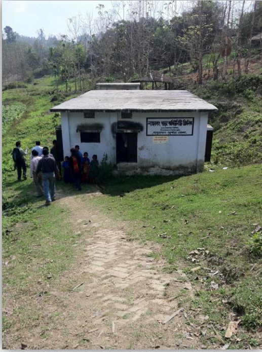
FIGURE 4-3 COMMUNITY CLINIC, BANDARBAN
