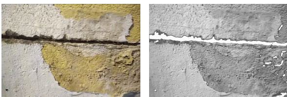
Figure 3: Example of original vs resulting image after flaw separation.
