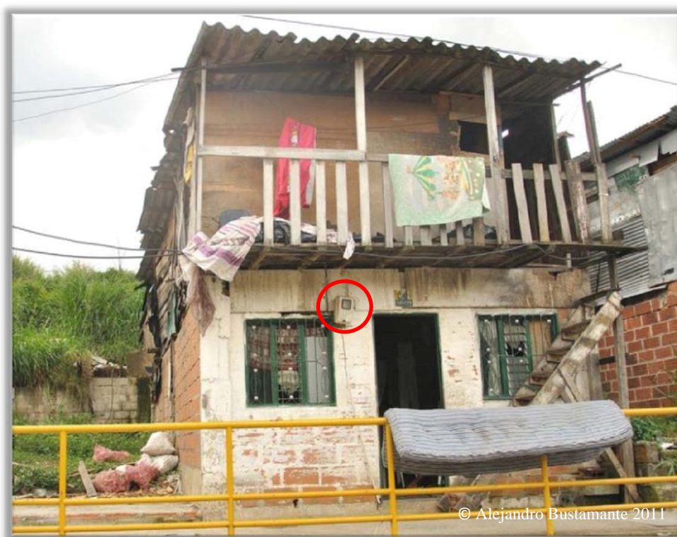
Figure 13: Informal dwelling in different stages of consolidation legally connected to the public electricity network, Medellin.
