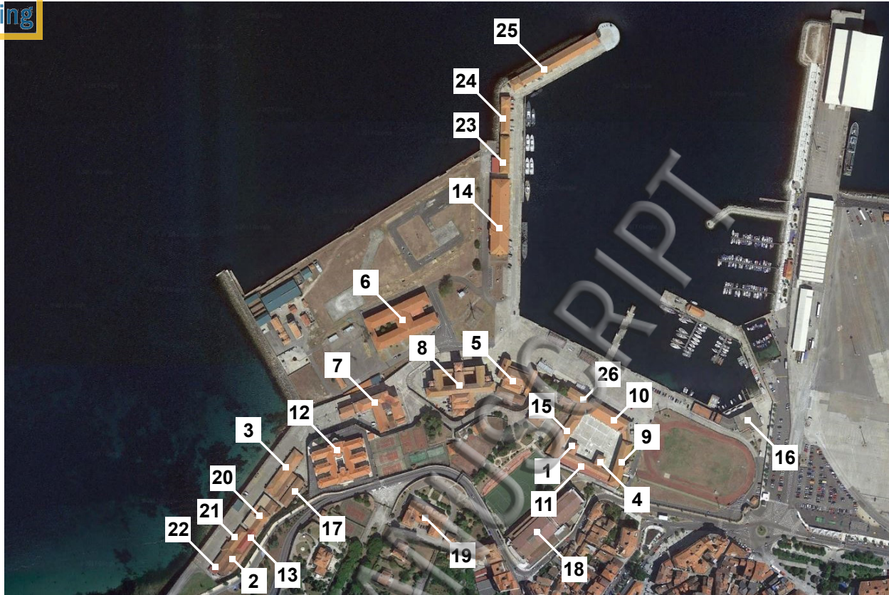
FIG. 2: Aerial photography of ENM ground facilities
