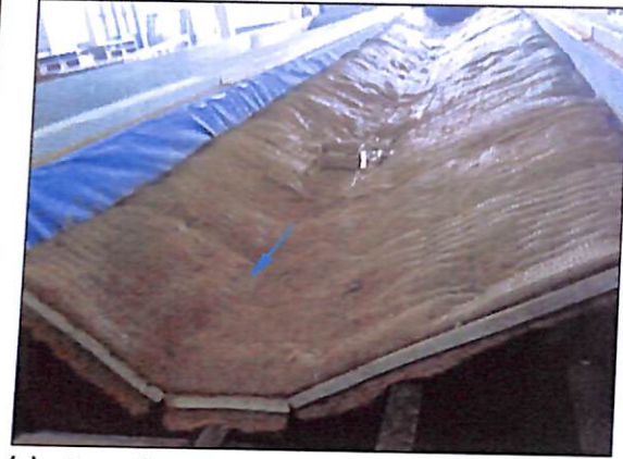
(c) Completion Works of Laying and Stapling TRM
