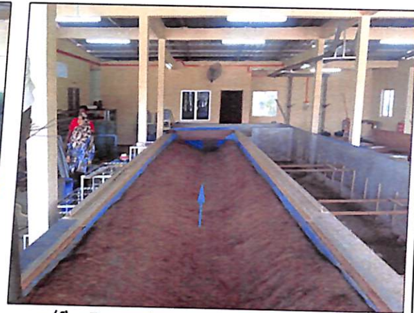
(f) Downstream of Earth Channel
