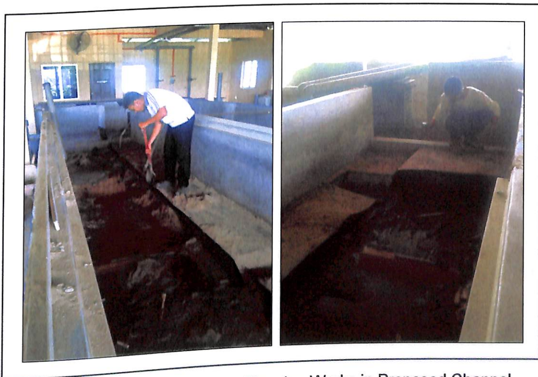
Figure 3.7: Dismantling and Cleaning Works in Proposed Channel
