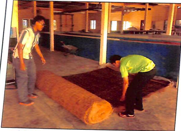
(a) Unroll the TRM for Laying Works
