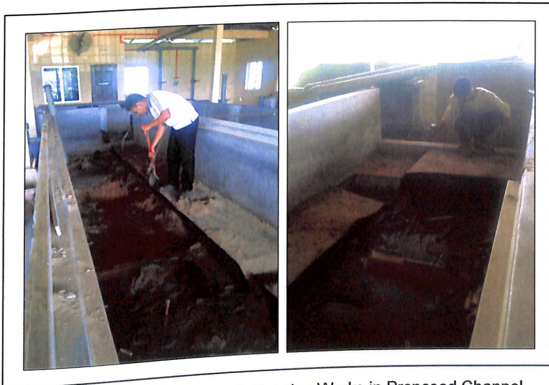
Figure 3.7: Dismantling and Cleaning Works in Proposed Channel
