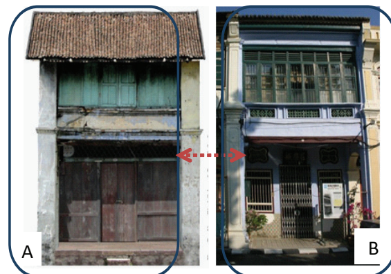
Figure 9: (A) Early Penang Style with timber and attap (B) Sun YatSen/ Southern Chinese Eclectic /Source: penangshophouse.com.my , 2015 Modified By Author
