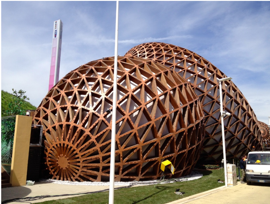
Figure 13: View from the outside
