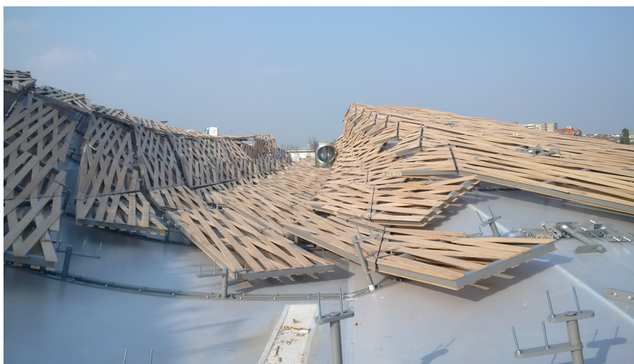
Figure 6: Membrane and bamboo installation
