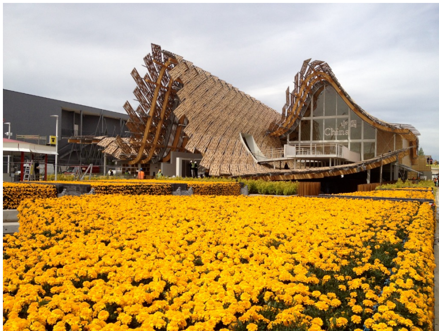
Figure 8: Pavilion with membrane cladding and bamboo panels
