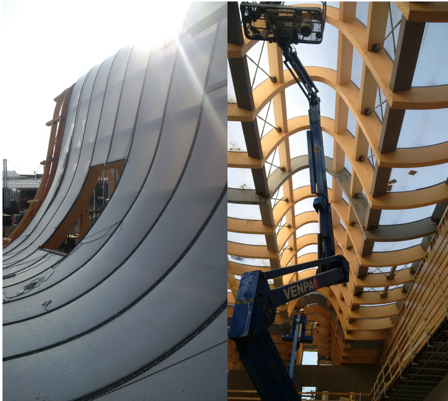
Figure 7: Membrane installation
