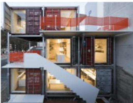
Figure 10: Office building out of sea containers [14]
