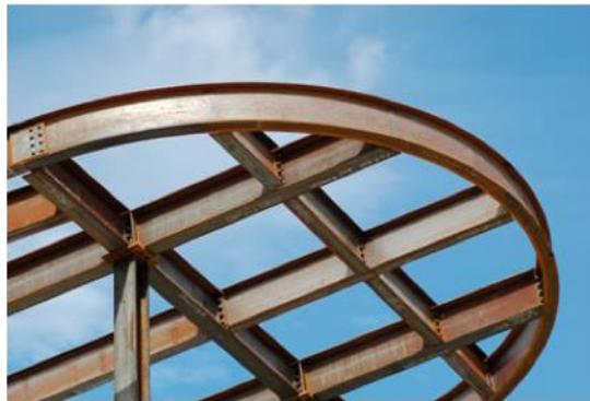
Figure 52: Example of a construction in the USA, I-profiles for the flooring structure [26]
