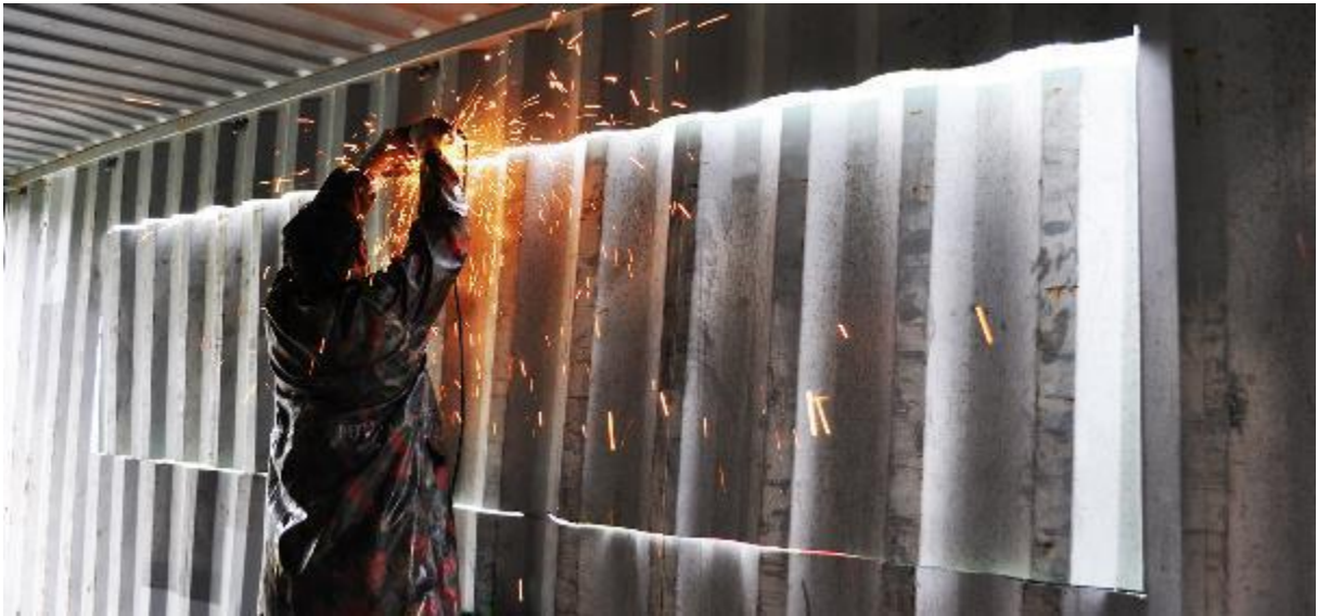
Figure 104: Cutting windows and doors [75]
