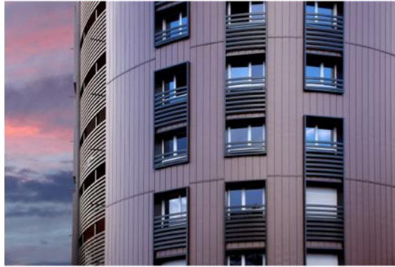
Figure 53: Bended zinc coil sheets as a finishing [27]
