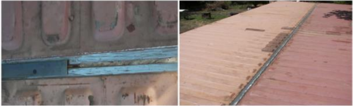
Figure 108: Welding the containers together [78]
