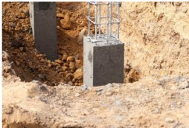
Figure 57: Metal reinforcements in foundation piles [35]
