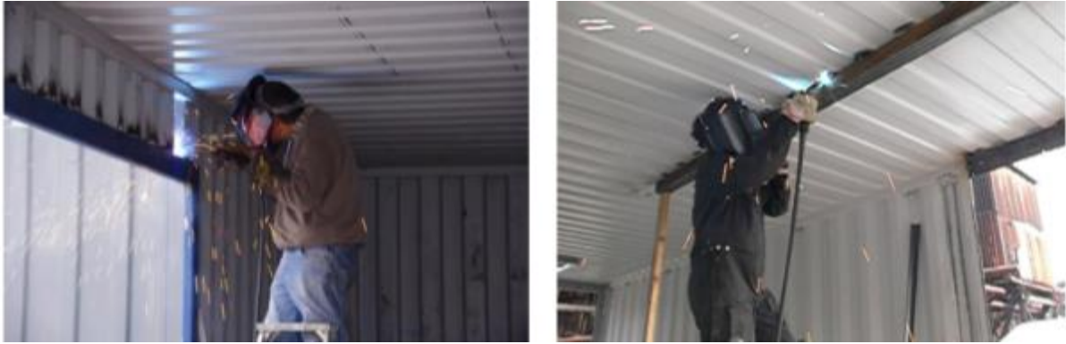
Figure 109: Welding window and door frames (left) [79] & reinforcements (right) [80]
