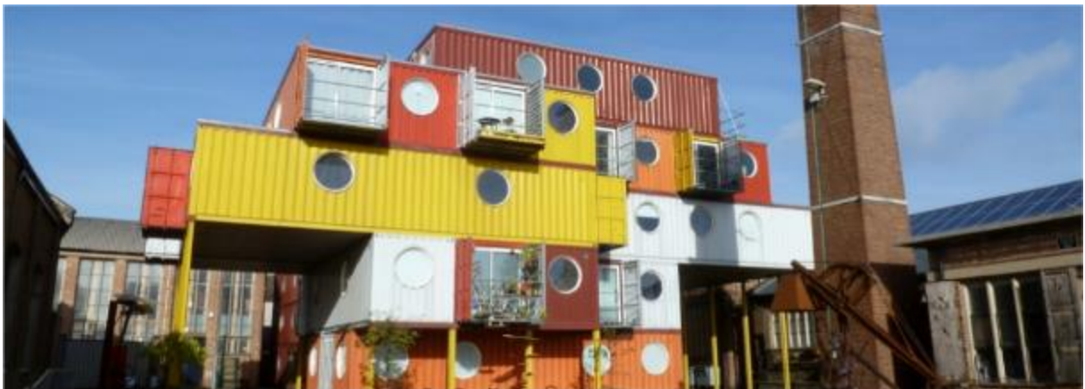
Figure 7: Container City in London [11]
