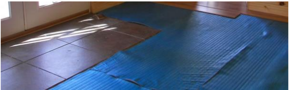
Figure 115: Non-breathable flooring underlayment [87]
