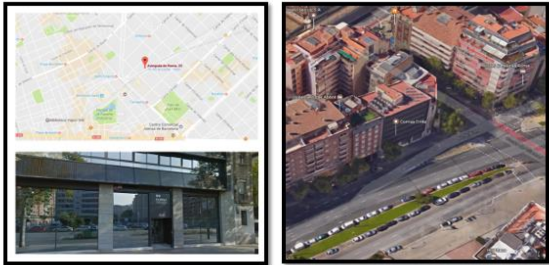
Figure 1. Left: Emplacement of COMSA Headquarters in Barcelona and main entrance. Right: 3D Google view of the building.
