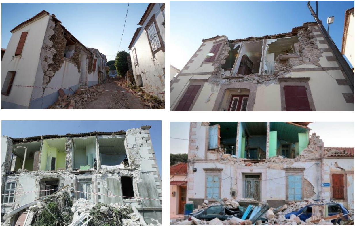
Figure 1.1 Out-of-plane collapses of traditional Unreinforced Masonry (URM) houses during the earthquake in Lesbos 2017
