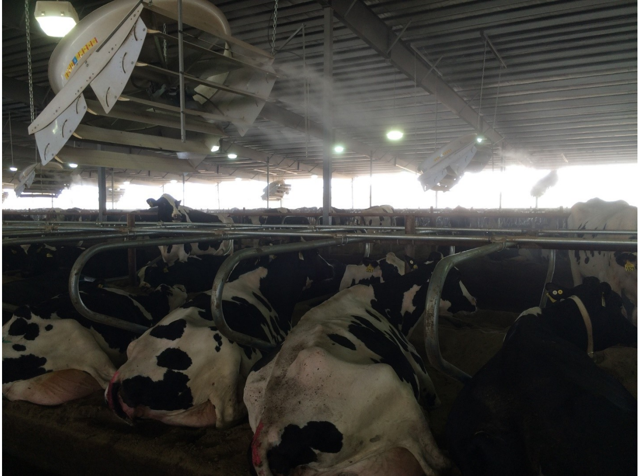
Figure 5.9 Photo showing the evaporative cooling system (ECV72 fans and fog) over the resting area in the tunnel-ventilated freestall barn.
