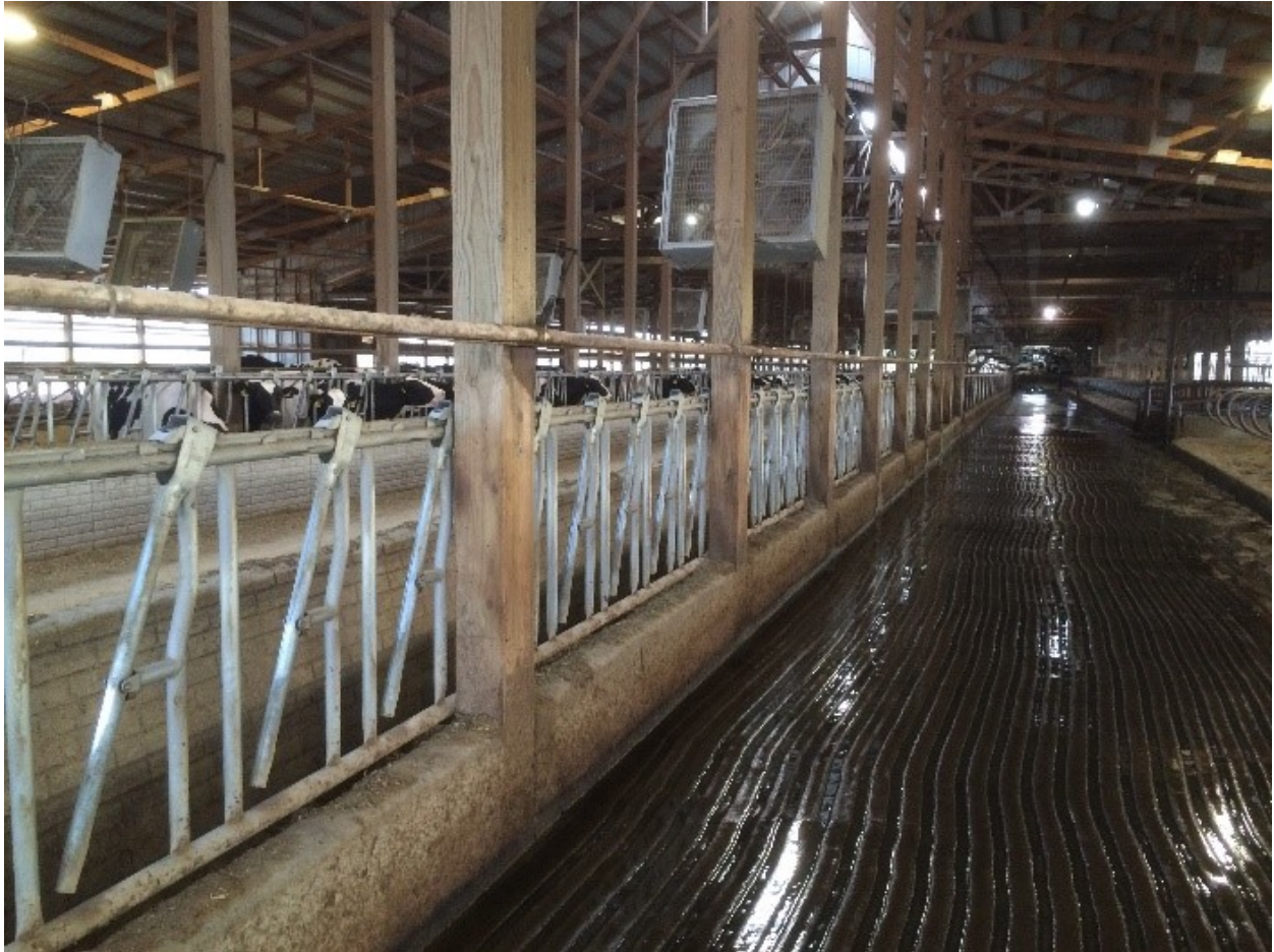
Figure 5.10 Photo showing the cooling system (feedline soakers with fans over the feedline) in the open-sidewall, conventional freestall barn. Fans were also located over the resting area.
