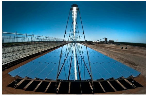
Figure 6. Linear Fresnel collector (LFC). Source: AREVA solar.
