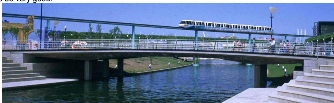
Figure 1. View of the structure.
