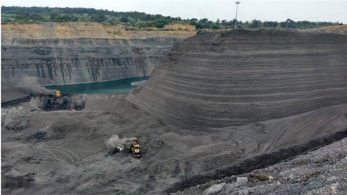
Figure 24 - Overview of Belpahar OCP (3)
