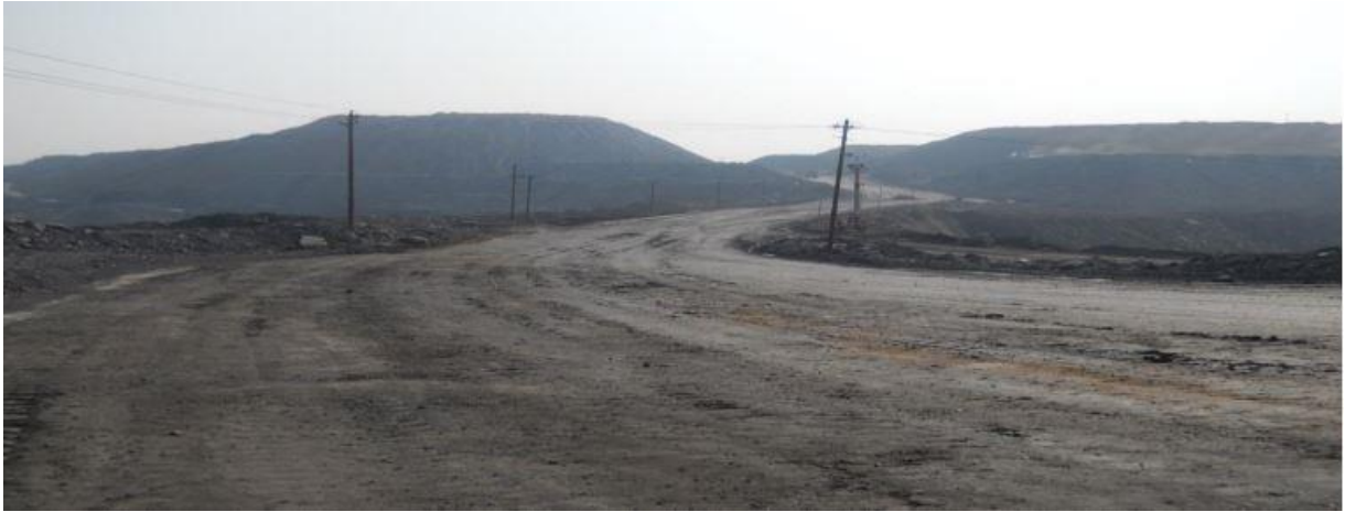
Figure 22 - Overview of Belpahar OCP (1)
