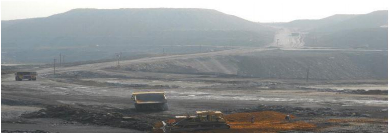
Figure 23 - Overview of Belpahar OCP (2)
