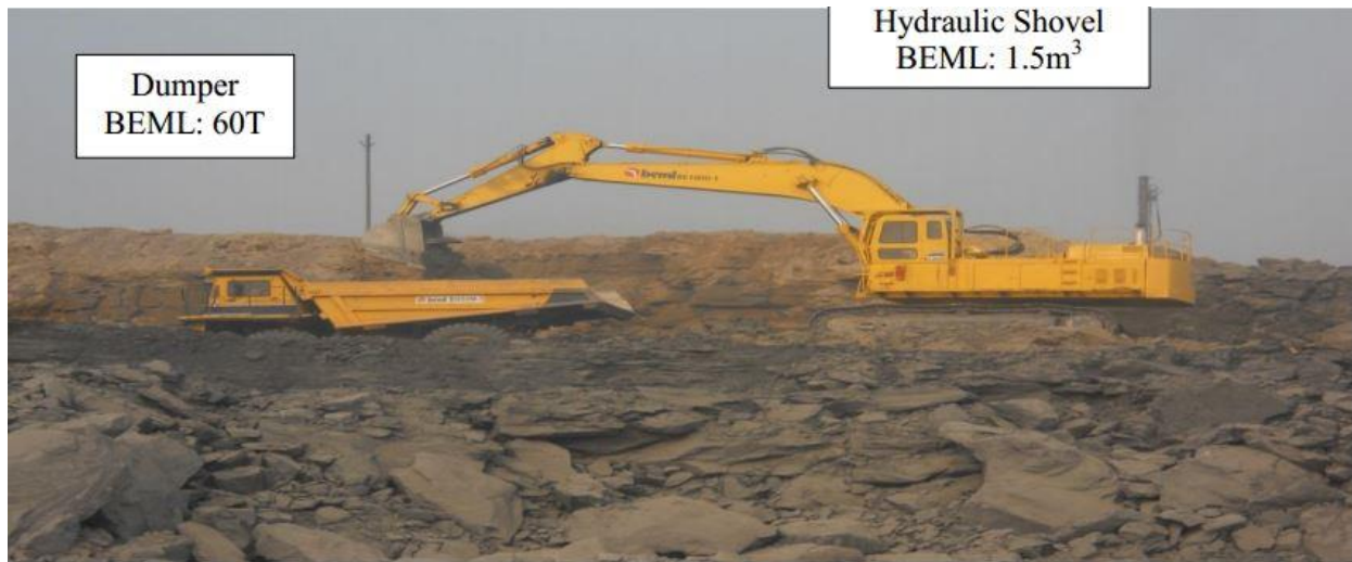
Figure 26 - Working of Shovel and Dumper
