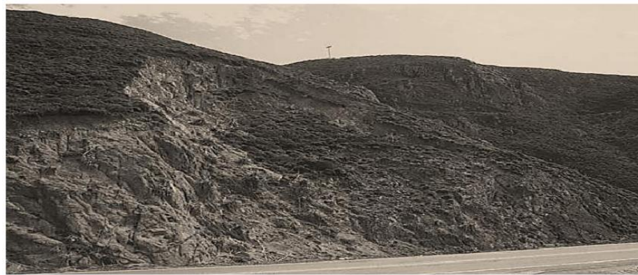
Figure 7 – Circular failure in highly weathered, granitic rock (on Highway 1, near Devil's Slide, Pacifica, California). (Source: Rock slope engineering, 4th edition by Duncan C. Wyllie and Christopher W. Mah,)
