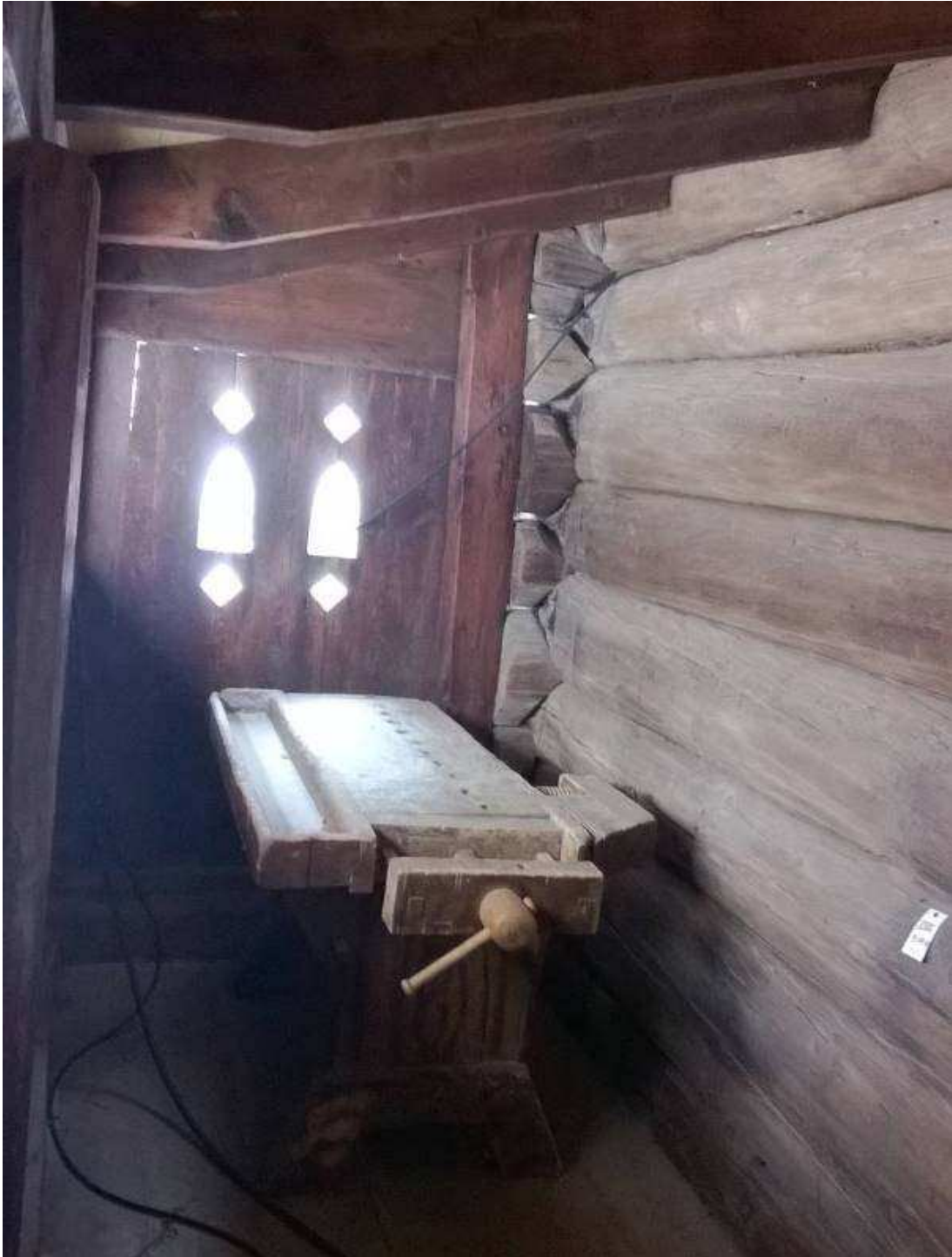
Figure 3: Svalgang of Hjeltarstua from 1763, recently placed in the Maihaugen Open Air Museum in Lillehammer (photo: Davidová 2016) shows the opportunity of indoor-outdoor environment including the range from social to climatic interaction while working actively.
