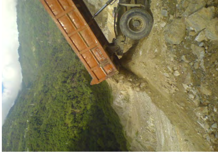
Picture b: Truck unloading debris on to the slope
