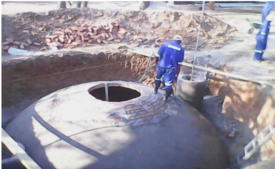
Fig. 1.1: Biogas digester of size 50 m 3 under construction (Rural Electrification Fund, 2015)
