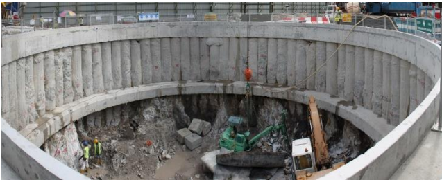
Figure 9 Circular shaft during excavation.
