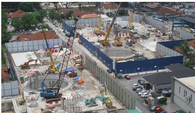
Figure 10 Overall view of the two completed TBM launching shafts (picture sourced from internet).
