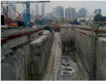
TRX Station (excavation in progress).
