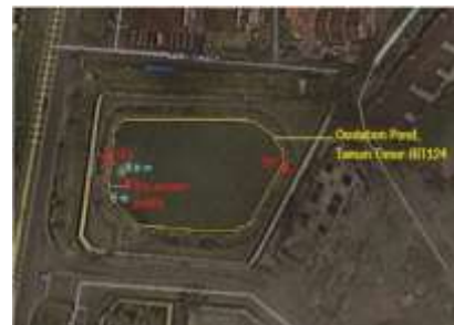
Figure 2 The aerial view of the oxidation pond at Taman Timor, Johor
