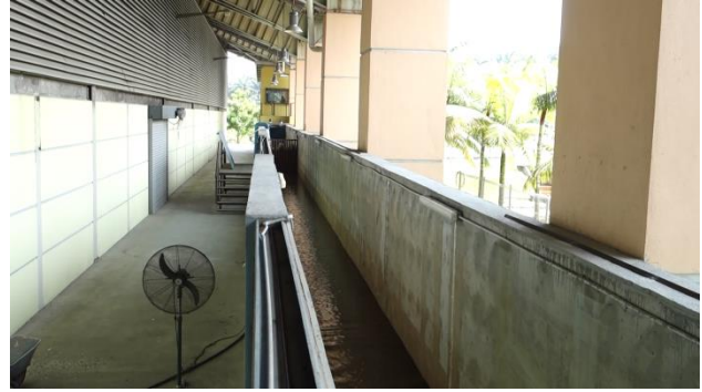
Figure 4 Flume facilities at NAHRIM
