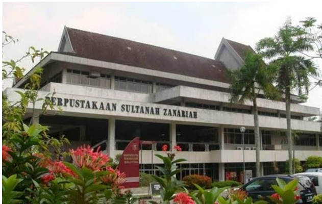
Figure 2 View of the library building
