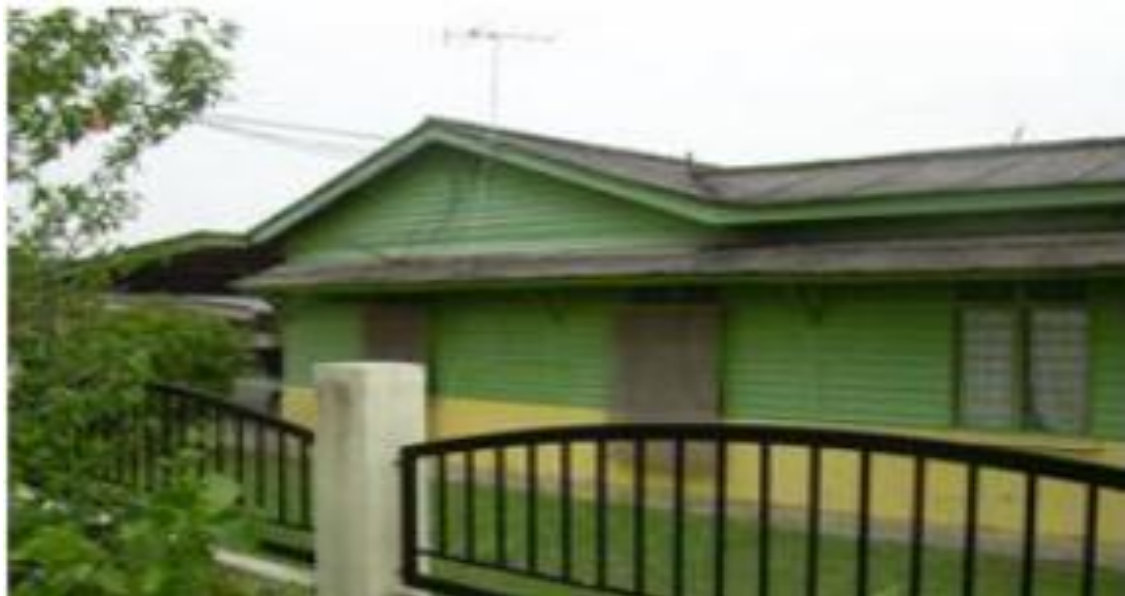
Figure 2.3: Typical Project Using Timber Forming System (Sufian, 2009)
