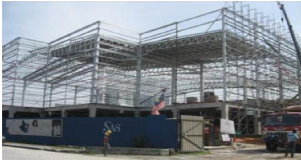
Figure 2.2: Typical Project Using Steel Framing System (Sufian, 2009)
