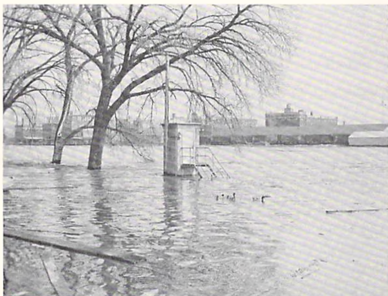
Figure 3. CONCRETE GAGE HOUSE ON CEDAR RIVER AT CEDAR RAPIDS, IOWA, AT PEAK OF FLOOD ON MARCH 31, 1961.
