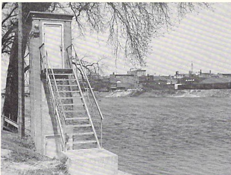
Figure 2. CONCRETE GAGE HOUSE ON CEDAR RIVER AT CEDAR RAPIDS, IOWA, DURING LOW FLOW.
