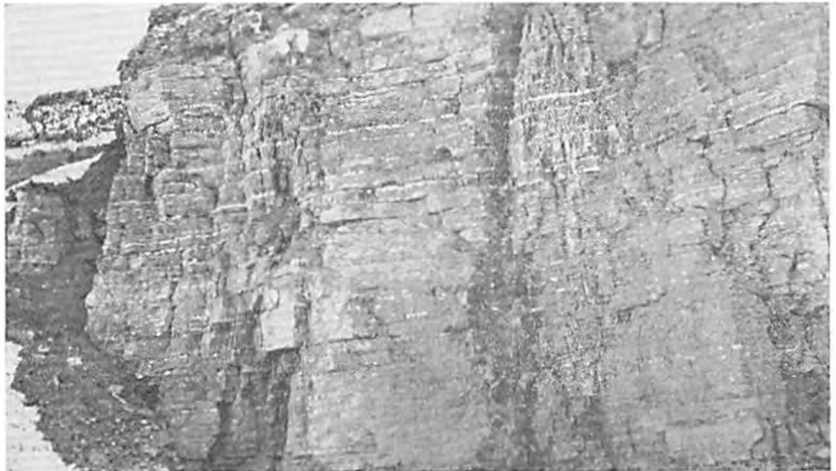
PLATE 9.—EXPOSURE OF THE KANKAKEE LIMESTONE IN A QUARRY (93-6-36P1Q) NORTHEAST OF VOLGA, SHOWING THE THIN-BEDDED AND NODULAR WHITE CHERT THAT IS CHARACTERISTIC OF THIS FORMATION.
