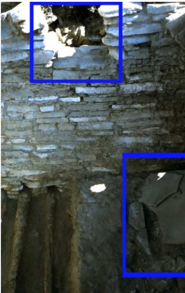
Fig. A.20: Photograph upper-storey Room 8b, showing: the east doorway (only known exterior doorway of the North Suite); the prepared clay floor (Surf 1) overlying intact secondary beams; and the Surf 1 hatchway and its in-situ cover in the southeast corner of the room.
