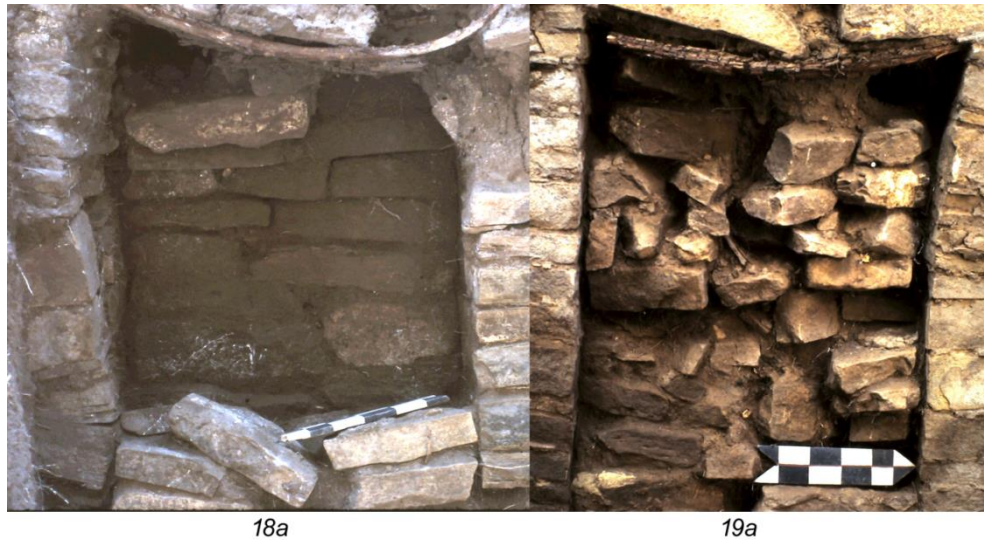
Figure A.7: Photographs of the distinctly different appearances of the masonry used to block the west (18a) and east (19a) sides of the 18a/19a doorway. The appearance of the 19a side is representative of plugged doorways observed at Wallace Ruin.
