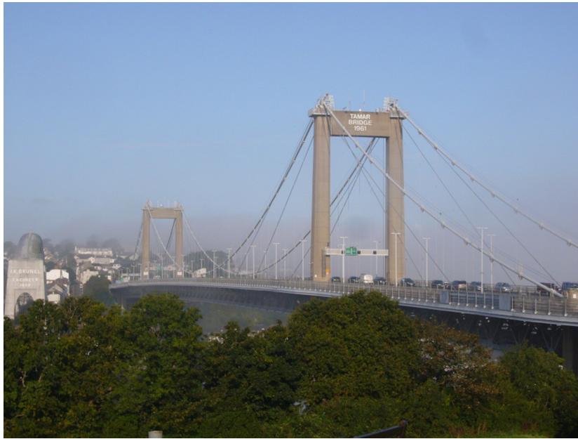
Fig. 1. The Tamar Suspension Bridge.
