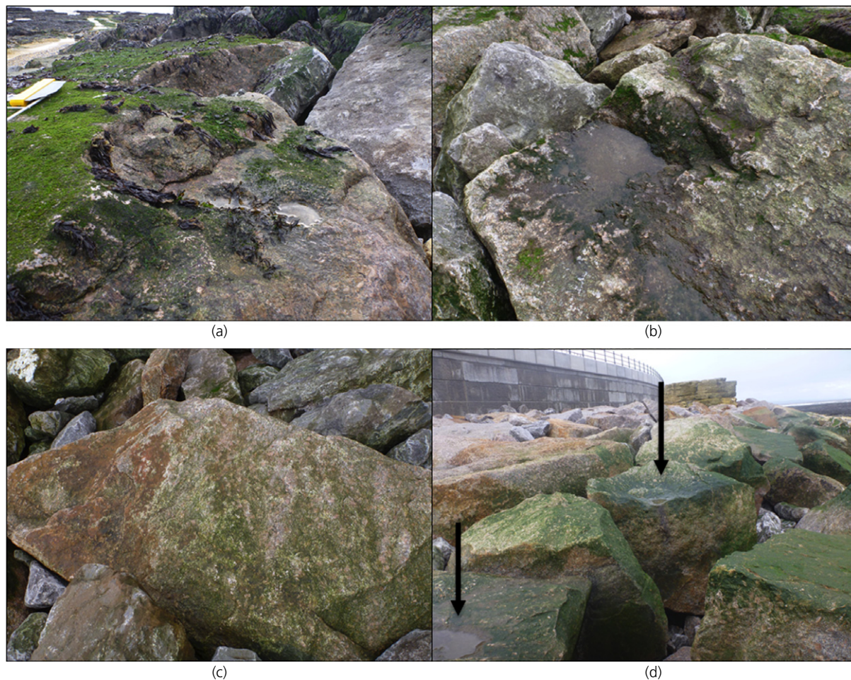
Figure 6. Passive enhancement of rock armour compared with partially enhanced rocks. (a) Positioning of a passively enhanced rock so that depressions are face-up. (b) Water-retaining capacity of passively enhanced rock. (c) Partially enhanced rock, with smooth, featureless surface and (d) rock revetment with two passively enhanced rocks in the foreground/centre (black arrows) separated by partially enhanced rocks. The rock shown in part (a) was installed during 2015 (colonisation data included in this paper) and the rocks shown in parts (b), (c) and (d) were installed during 2016, showing differences in ecological colonisation
