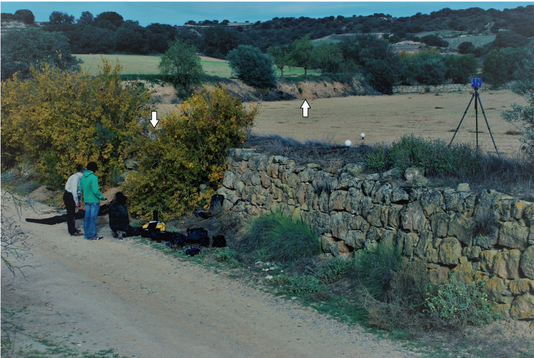
Figure 3. Fieldwork on the Balaguer-Castelló road (looking north-west). Arrows indicate the location of profiles taken from the stone-faced check-dam in the foreground and the earth bank in the background, which delimits the gently-sloping terraced field behind. Photo: Sam Turner, November 2014.
