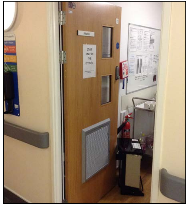
Kitchen door: Ward A
