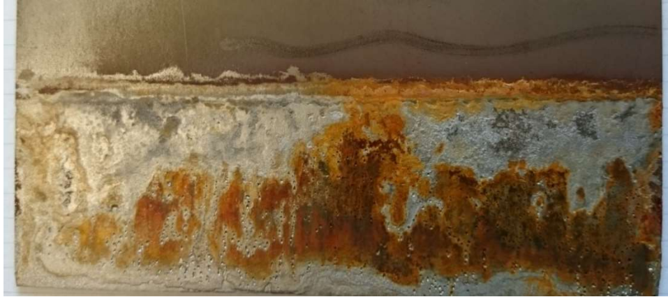
Figure 5-24 – Accelerated Sample with Excessive Corrosion
